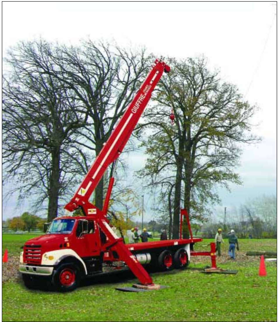
Proper crane use can greatly increase efficiency and safety in removal operations – provided both the tree crews and crane operator are well trained.
